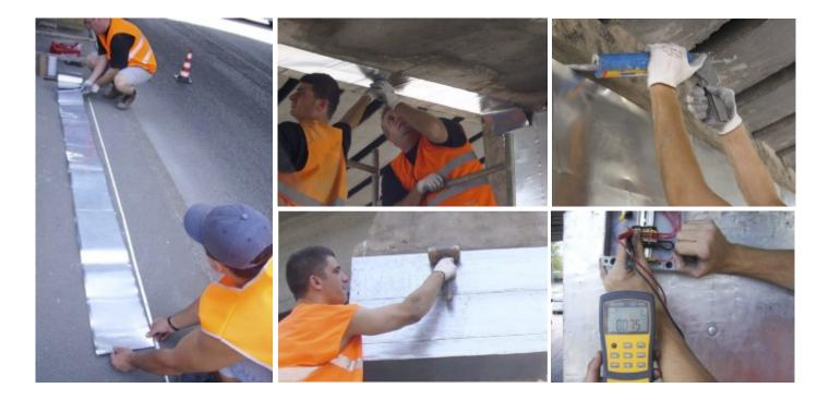
After cutting the ZLA into the appropriate length can be applied onto a cleaned concrete surface by hand application. Old concrete surfaces must be structurally sound with any unsound areas being repaired prior to the installation of ZLA. Laitance and other surface contaminants also need to be removed.
